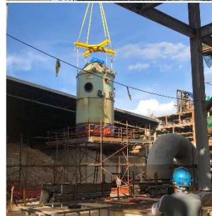
H 2 S Scrubber Tank Bottom Half Removal
