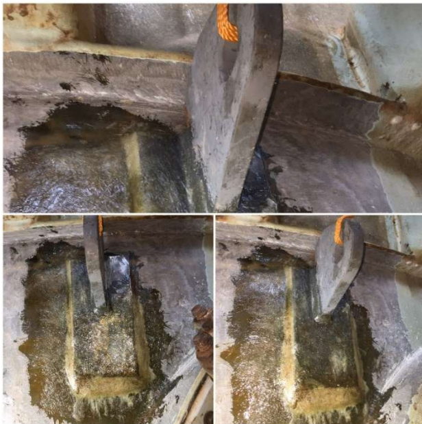
Lifting Lug Lamination to Scrubber Tank Shell
