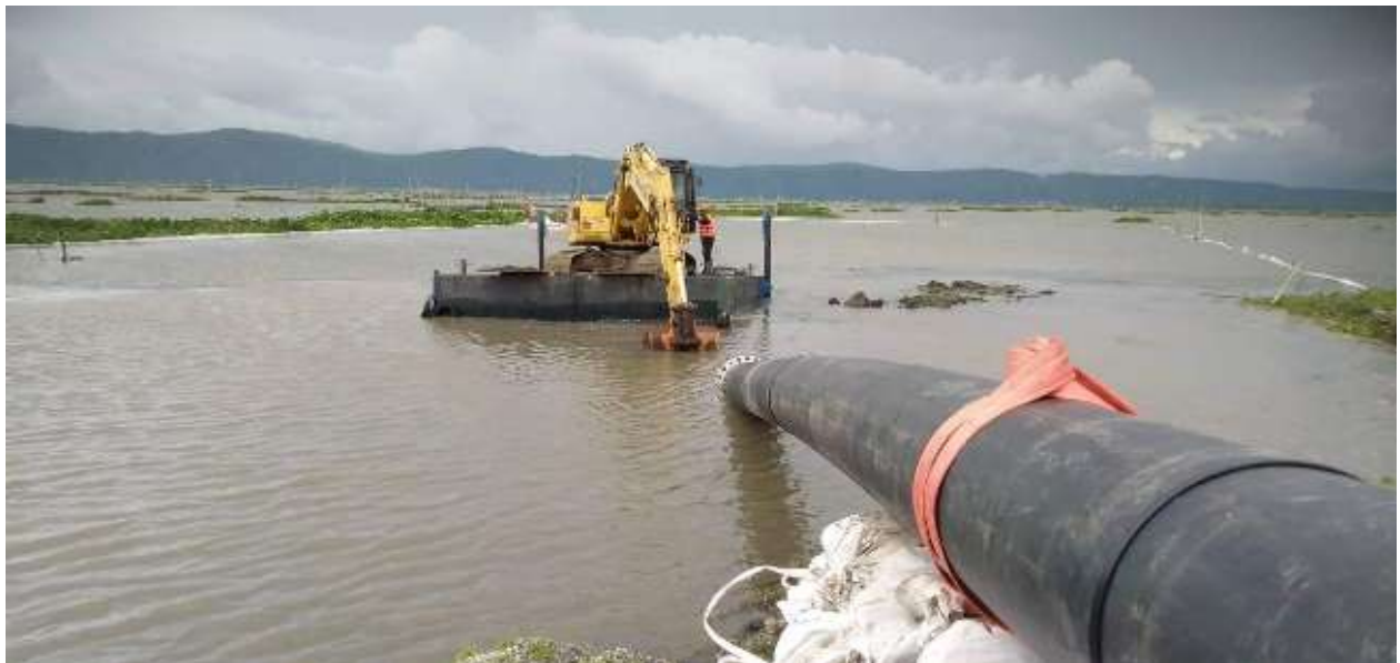
OFFSHORE PIPE TRENCH EXCAVATION
