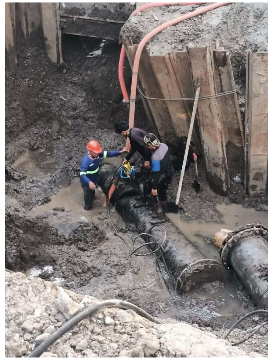
INSTALLATION OF THE MODIFIED ROUTING FOR 600 MM DIA. UNDERGROUND OUTFALL PIPE
