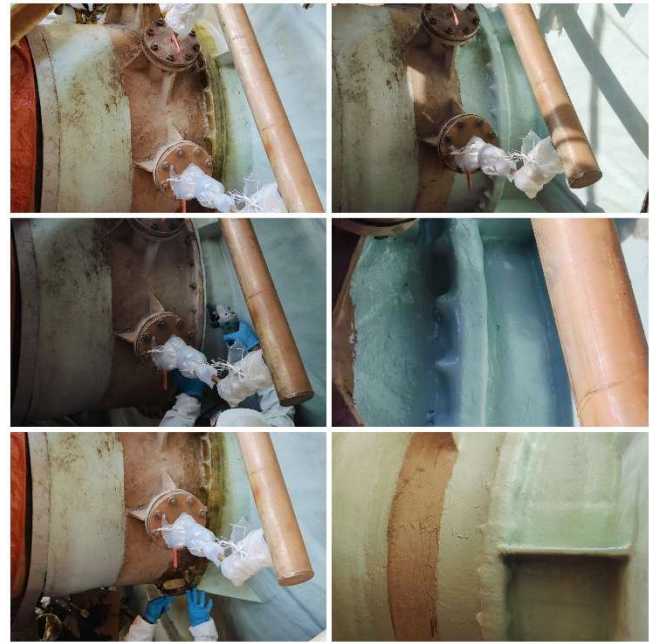
Gas inlet Flange Connection Lamination
