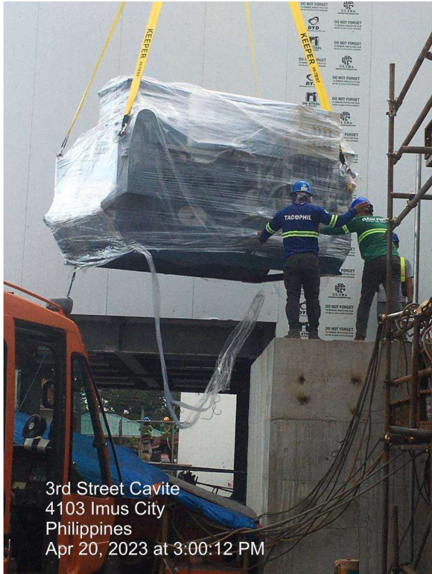
BELT PRESS INSTALLATION AND POSITIONING
