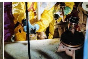
H 2 S Scrubber Tank Bottom Half Removal
