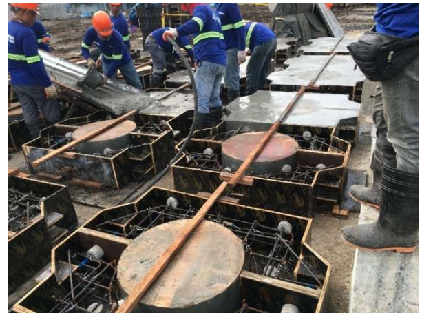
HDPE PIPE CONCRETE BALLAST (SINKER) FABRICATION
