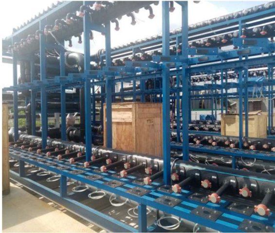
UF SKID POSITIONING & INSTALLATION
