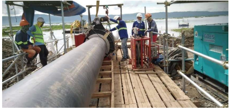
600 & 800-MM DIAMETER HDPE PIPE JOINTING (BUTT FUSION WELDING)
