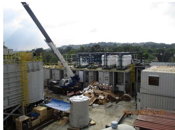
EQUIPMENT AND SKIDS INSTALLATION
