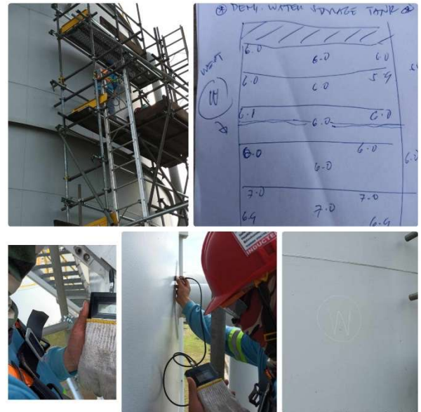
Steel Tank Wall Thickness inspection by UTZ
