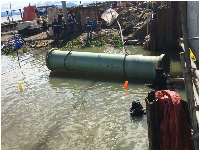
GRP PIPE SPOOL FINAL TIE-IN UNDERWATER INSTALLATION
