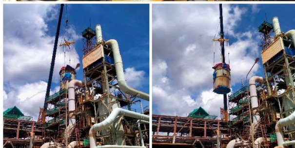
H 2 S Scrubber Tank Upper Half Removal
