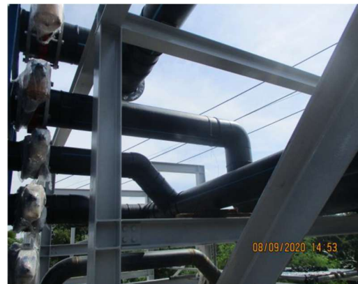
INTERCONNECTION PIPE FABRICATION AND INSTALLATION
