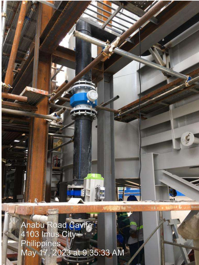
FABRICATION AND INSTALLATION OF TANK PIPING SYSTEM
