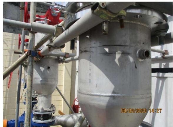
PUMP SUCTION AND DISC. PIPE INSTALLATION
