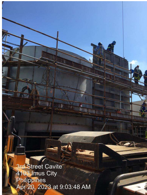
ON SITE ASSEMBLY OF STEEL CLARIFIER TANKS (HYDRO-PAQ)
