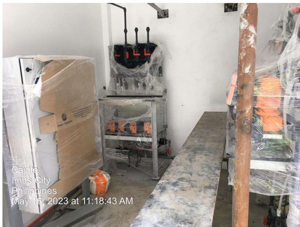
CHEMICAL PUMP SKID INSTALLATION
