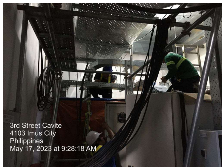
MCC & PLC PANEL BOARD POSITIONING, INSTALLATION AND CABLE ROUTING & TERMINATION
