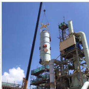
H 2 S Scrubber Tank Upper Half Removal
