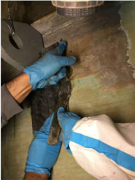
Lifting Lug Positioning to Scrubber Tank Shell
