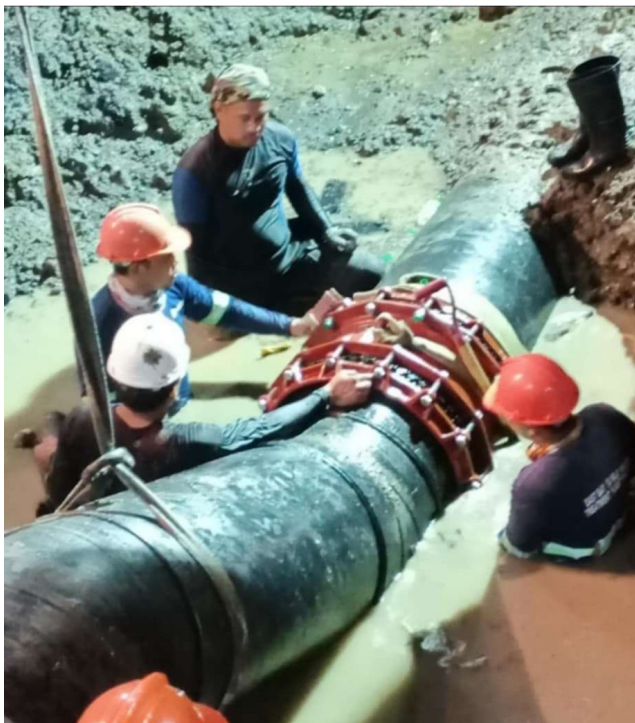
INSTALLATION OF THE MODIFIED ROUTING FOR 600 MM DIA. UNDERGROUND OUTFALL PIPE
