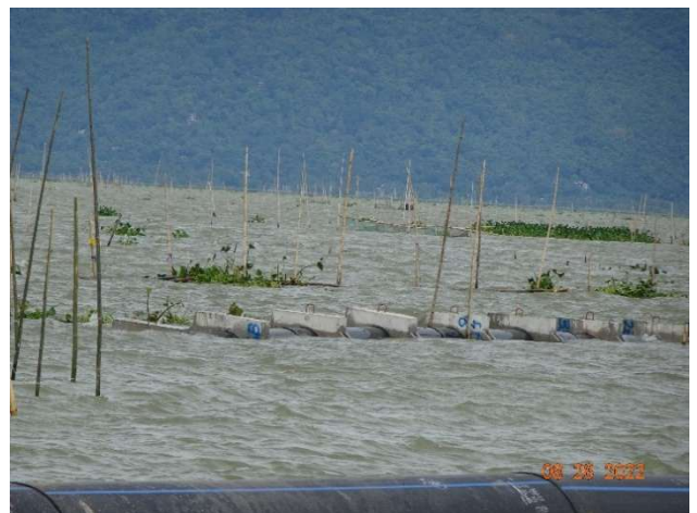
HDPE PIPE SINKING
