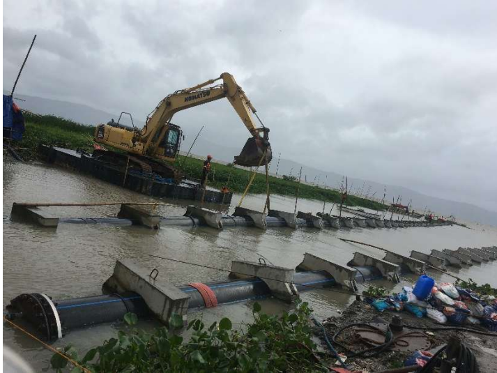
INTAKE PIPE POSITIONING, INSTALLATION AND ALIGNMENT
