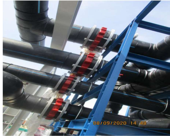
HDPE PIPE AND VALVE TIE-IN INSTALLATION
