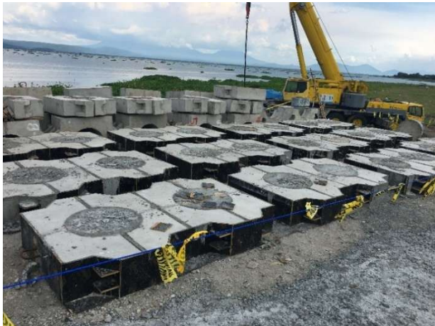
HDPE PIPE CONCRETE BALLAST (SINKER) FABRICATION
