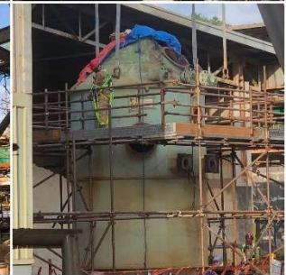
H 2 S Scrubber Tank Bottom Half Removal
