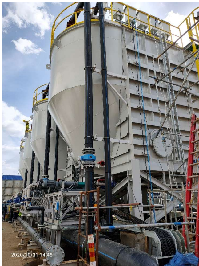
CLARIFIER TANK PIPING FABRICATION & INSTALLATION
