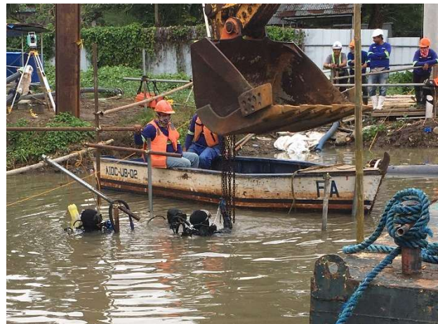
GRP PIPE SPOOL FINAL TIE-IN UNDERWATER INSTALLATION
