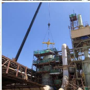
New H 2 S Scrubber Tank Installation
