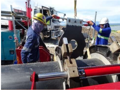
600 & 800-MM DIAMETER HDPE PIPE JOINTING (BUTT FUSION WELDING)
