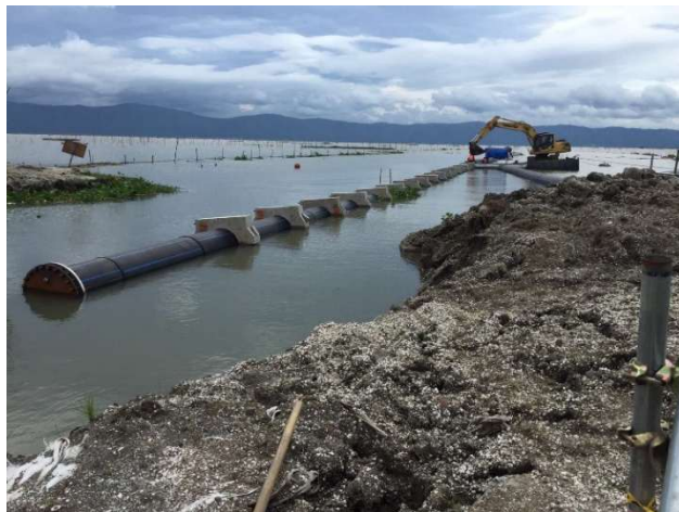
HDPE PIPE SINKER INSTALLATION
