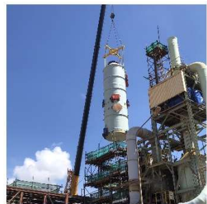
H 2 S Scrubber Tank Upper Half Removal
