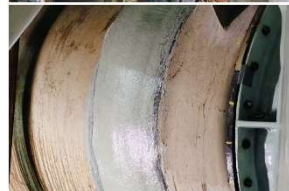
Gas Inlet Ducting Cutting and Lamination
