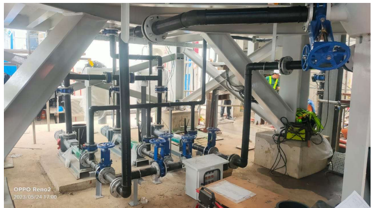
SLUDGE PUMP & PIPING SYSTEM INSTALLATION
