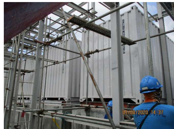
CHEMICAL TANK SKID INSTALLATION
