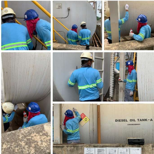
Steel Tank Visual Inspection for Corrosion
