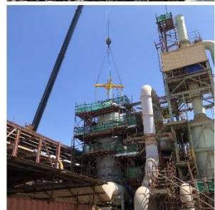
New H 2 S Scrubber Tank Installation
