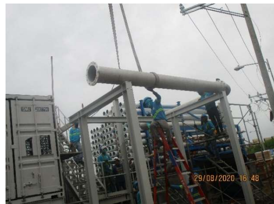
PUMP SUCTION AND DISC. PIPE INSTALLATION
