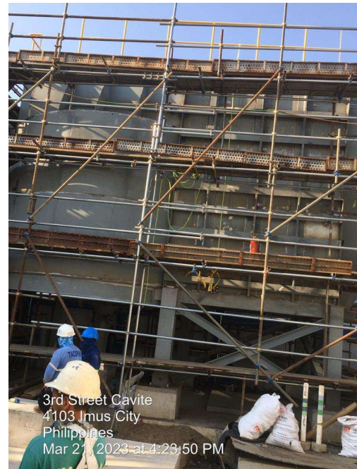
ON SITE ASSEMBLY OF STEEL CLARIFIER TANKS (HYDRO-PAQ)
