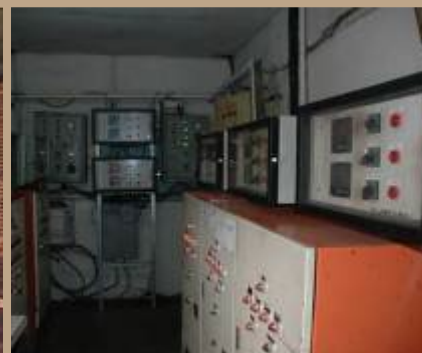
Kiln dry : 7 chambers up to 350m 3 , electronic panel, timber moisture content controlled regularly.
